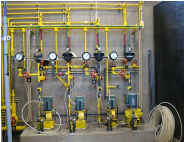
*Pipes and gauges are part of a water system control room. Operators monitor various gauges to ensure proper pressure is maintained and the appropriate mix of chemicals is added to the system to help maintain safe and adequate service.*
