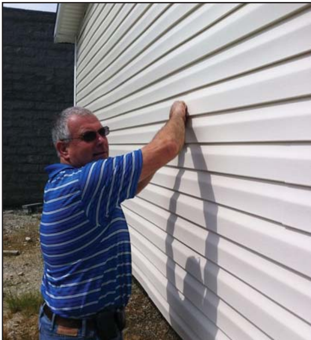
PSC Inspector David Freeman conducts an on-site inspection.
