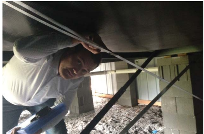
PSC Inspector Nate Haldiman examines anchor straps.
