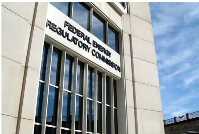
FERC building, Washington, DC
