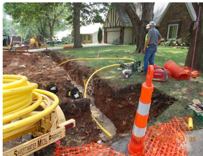
Natural Gas Pipeline Safety inspection in Springfield.
