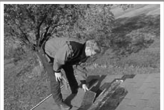
PSC Manufactured Housing Inspector Ronnie Mann examines roof damage on a manufactured home.
