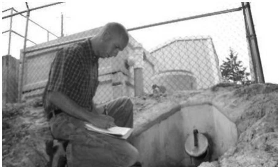
PSC employee Jerry Scheible inspects the quality of effluent leaving an extended aeration wastewater treatment plant.
