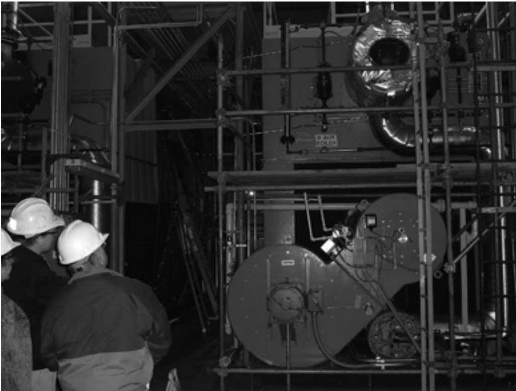
A photo of the turbine deck and auxiliary boiler system at the Hawthorn 5 power plant operated by Kansas City Power & Light.
