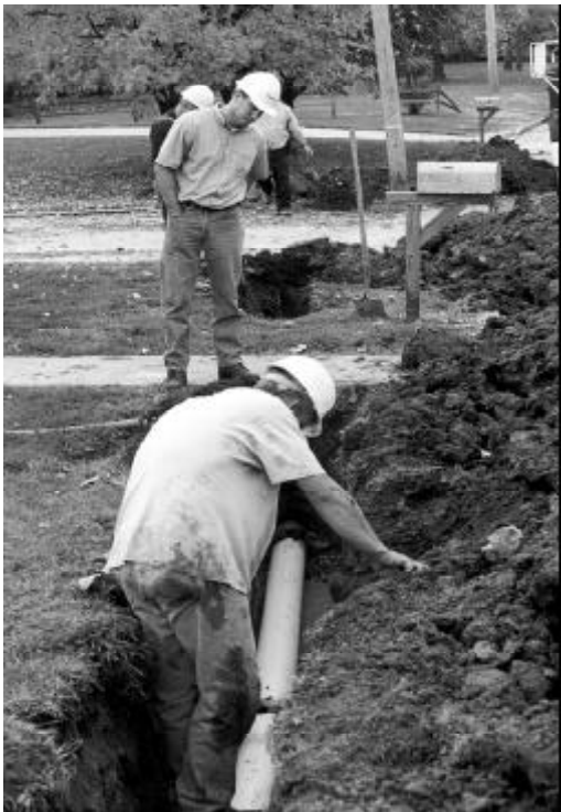
Workers for AmerenUE install state-of-the-art plastic natural gas pipeline as part of a replacement program. The new pipe is expected to eliminate corrosion problems underground.
