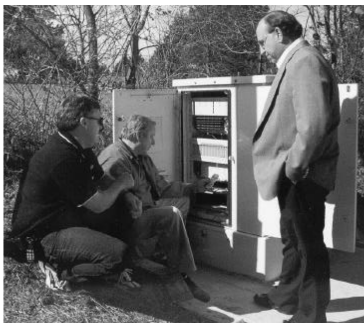
PSC staff inspect a "Remote Terminal" unit belonging to Kingdom Telephone Company near New Bloomfield, MO. Pictured left to right: Ron Whanger, Facilities Manager-Kingdom Telephone Company, and PSC Utility Operations Technical Specialists Mick Johnson and Larry Henderson.
