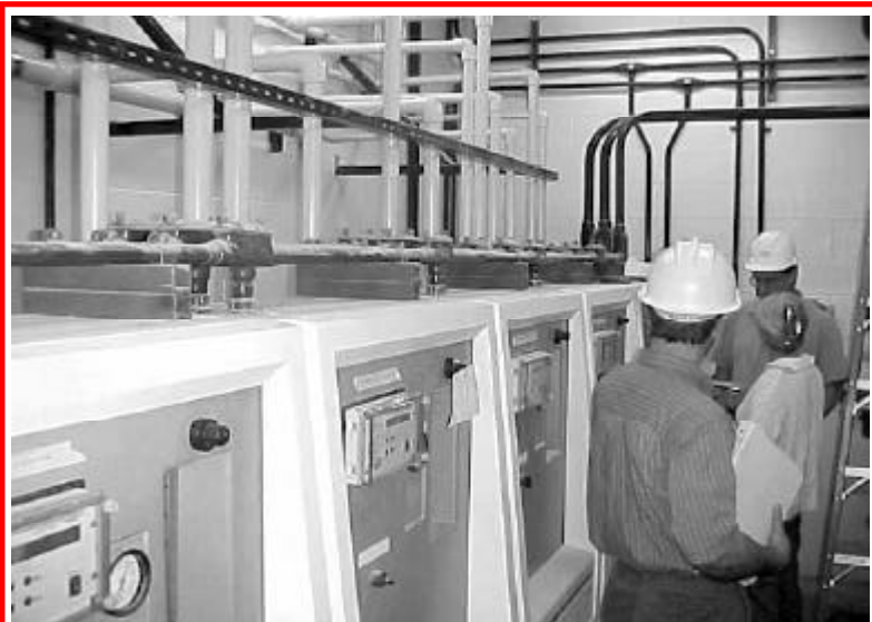
PSC Staff members inspect chlorine disinfection flow controllers at a Missouri water treatment facility.
