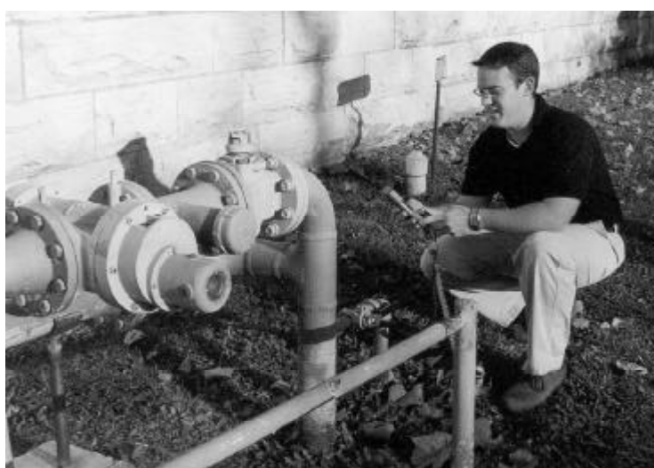
Energy Department Utility Engineering Specialist Greg Macias takes a cathodic protection reading at a natural gas regulator station. The reading measures pipeline voltage potential, which is used to help mitigate corrosion.
