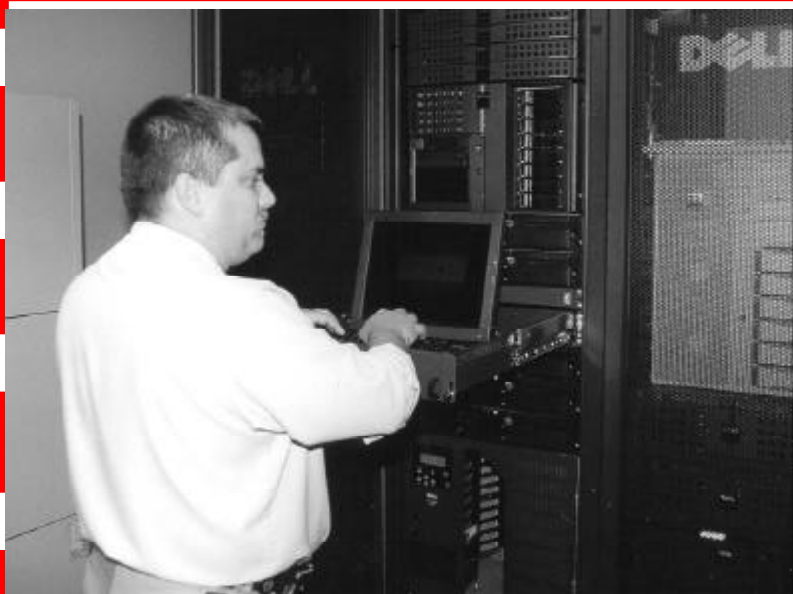
Todd Craig, Manager of the Information Services Department, is responsible for the engineering and maintenance of the PSC fiber-channel Storage Area Networks.
