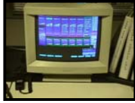
CRT Tele / Radio Switching
