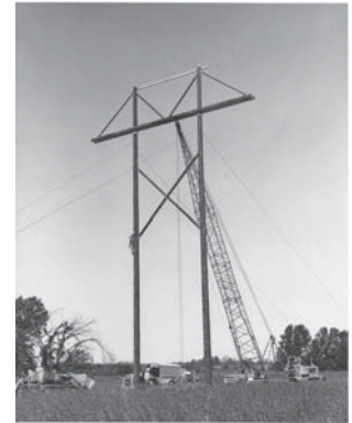
Union Electric transmission tower, 1965.
