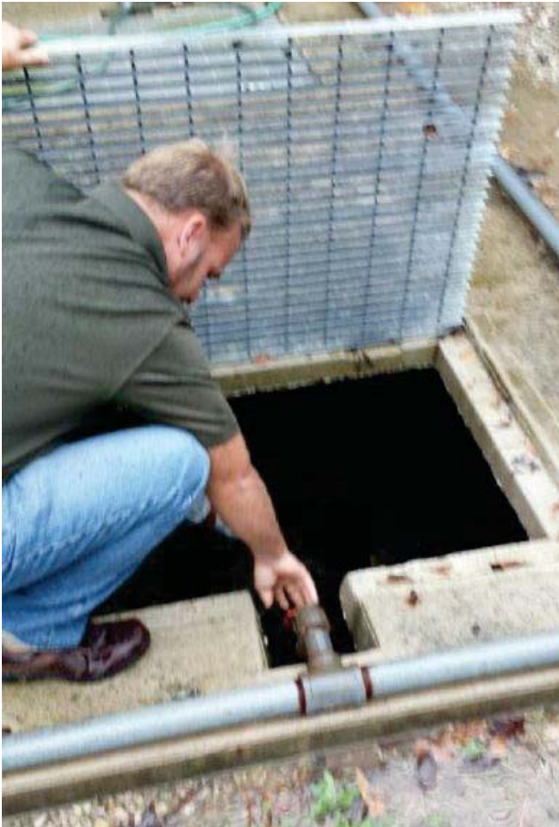
PSC Staff member Aaron Archer performs an on-site inspection.
