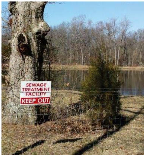
A sewage treatment lagoon.
