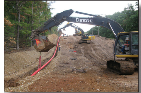
Excavation and installation of a gas line in southwest Missouri.
