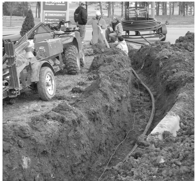
Workers install a two-inch plastic main near Lebanon.
