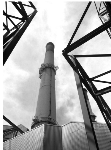
New construction at the Iatan 2 plant near Weston.
