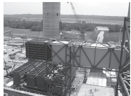
Work continues on the new Iatan 2 power plant near Weston. The plant is being constructed by Kansas City Power & Light Company.
