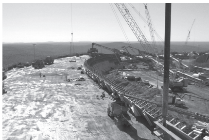
AmerenUE continues to work on rebuilding its Taum Sauk Pumped Storage project after a 2005 incident.
