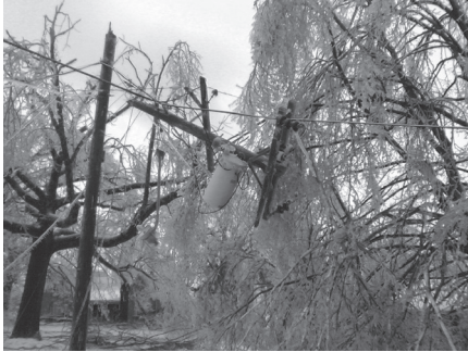
This photo shows some of damage the 2007 ice storm caused to the service territory of The Empire District Electric Company.
