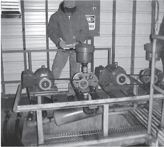
PSC staff member Jerry Scheible inspects a motor and blower assembly on a mechanical sewer treatment plant.
