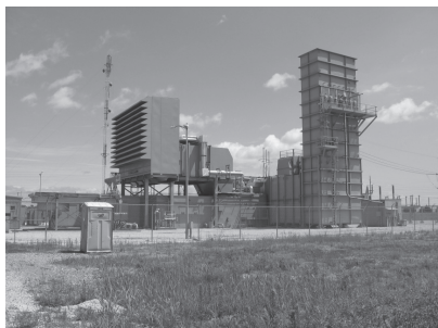
A natural gas fired turbine facility.
