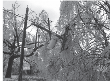
An ice storm in January caused massive damage in southwest Missouri. Photo courtesy of The Empire District Electric Company.
