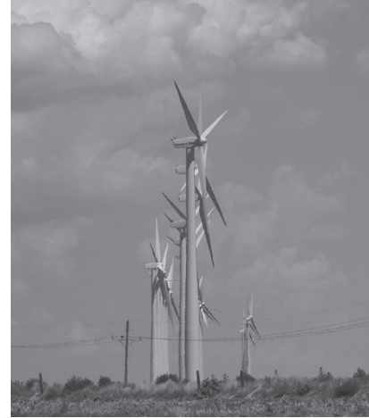
Part of the Gary County wind farm operated by Aquila near Dodge City, Kan. The blades are 67 feet long.
