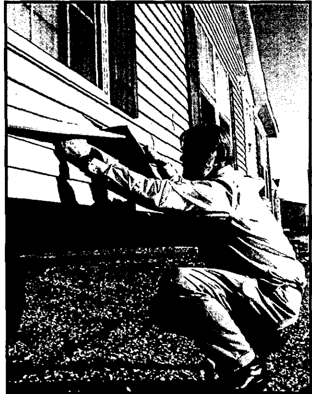
Gene Winn, Manufactured Housing Inspector/Supervisor, inspects the siding installation on a new manufactured home.
