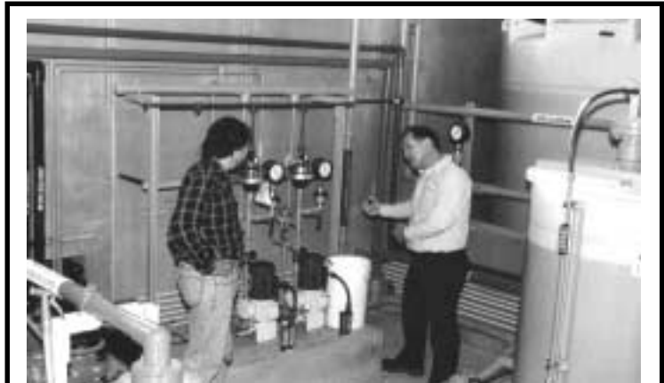
PSC Staff engineer Martin Hummel (left) and Missouri-American Water Company Production Manager Steve Ridenhour discuss the water treatment processes of a company water plant chemical room.
