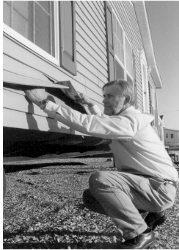
Gene Winn, Manufactured Housing Inspector/Supervisor, inspects the siding installation on a new manufactured home.
