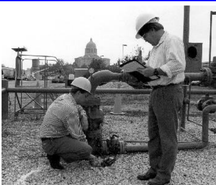
Gas safety specialists John Kottwitz (left) and Greg Williams take a cathodic protection reading at a regulator station. The reading measures pipeline voltage potential, which is used to help mitigate corrosion.
