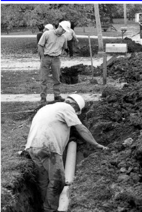
Workers for AmerenUE install state-of-the-art plastic natural gas pipeline as part of a on-going replacement program. The new pipe is expected to eliminate corrosion problems underground.
