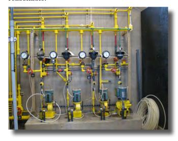
Pipes and gauges are part of a water system control room. Operators monitor various gauges to ensure proper pressure is maintained and the appropriate mix of chemicals is added to the system to help maintain safe and adequate
