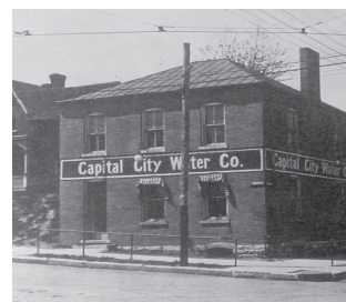
Capital City Water Co. in Jefferson City was organized in 1888. By 1938, it served about 4,000 customers.
