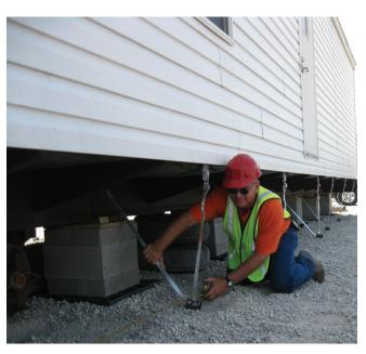
Ronnie Mann, a PSC Manufactured Housing Field Inspector, inspects the installation of the anchors under a FEMA Home at the Joplin Airport Site.
