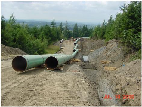
Figure 1 Transmission pipeline construction in the Northwest
