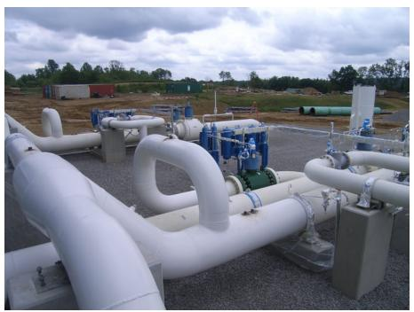
Figure 2 Regulation and Measurement Station
