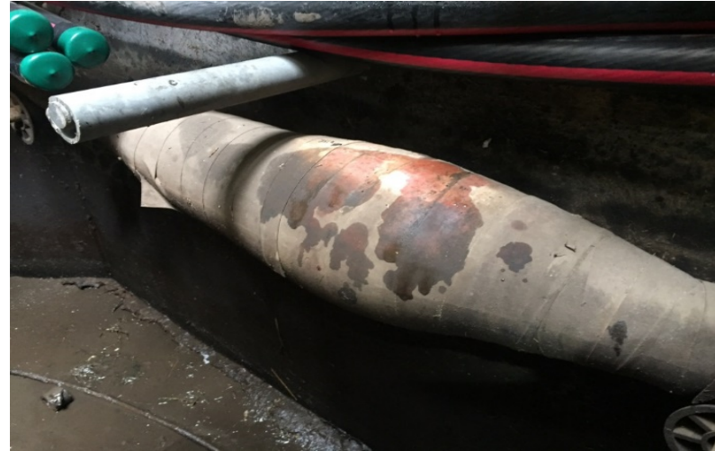
Paper Insulated Lead Cable (PILC)
